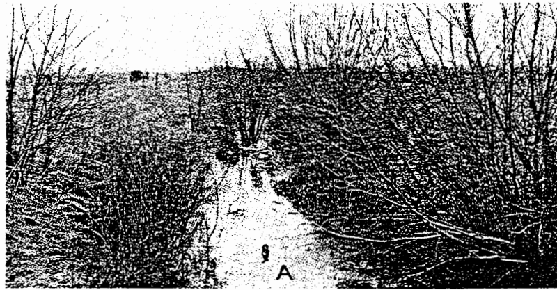
Two Mile Slough Dredged Channel near Sadorus, Illinois. Approximate bottom width 15 feet. Picture taken April 1925.
