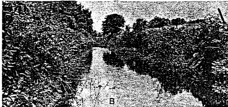
East Lake Fork Dredged Channel near Ivesdale, Illinois. Approximate bottom width 15 feet. Picture taken July 1927.
