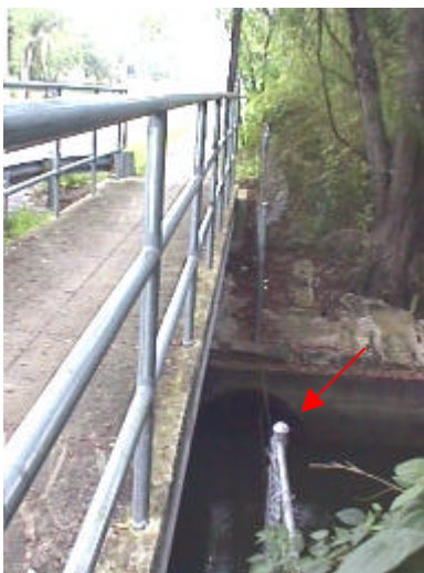
Figure 7-2. Curiosity Creek at Country Club Drive looking east. Note red arrow pointing to 60” culvert at bottom of photo which discharges untreated stormwater runoff (from Florida Avenue) directly to the creek.
