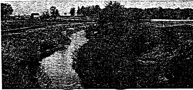
Kaskaskia River Dredged Channel near Sadorus, Illinois. Approximate bottom width 15 feet. Picture taken May 1926.
