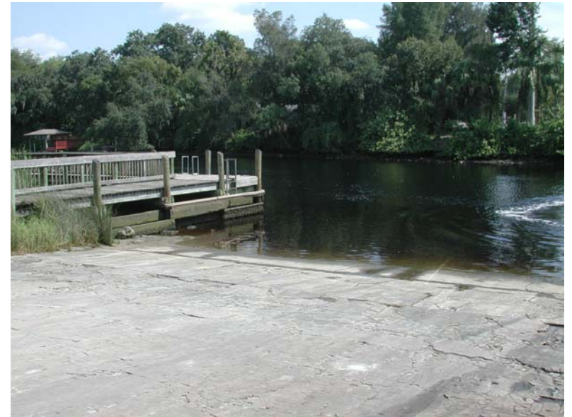
Figure 9 - Wide boat ramp launch
