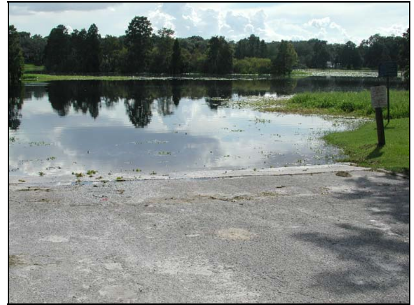
Figure 14 - Boat ramp at water's edge
