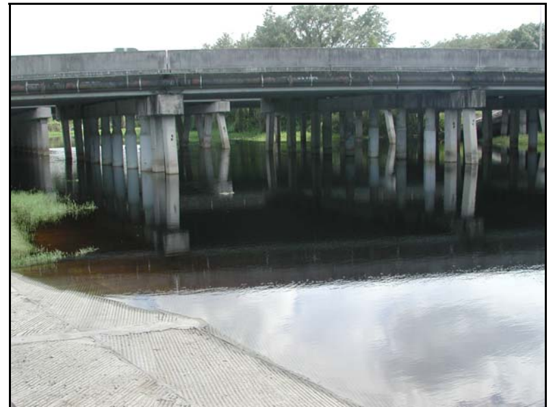
Figure 3 - Side view of the boat ramp next to bridge on Fowler Ave.
