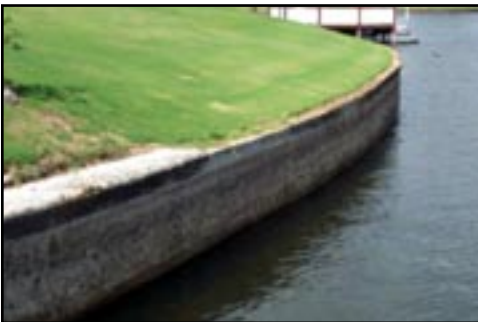
The concrete wall around the lake - low levels in June 2002 (USF)
